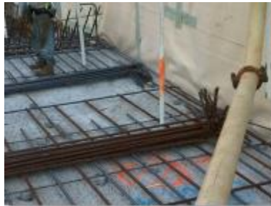
Dewatering system with temporary pipe penetrations.
